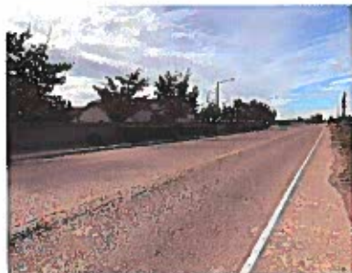
Temperance Avenue south of Adams Avenue
